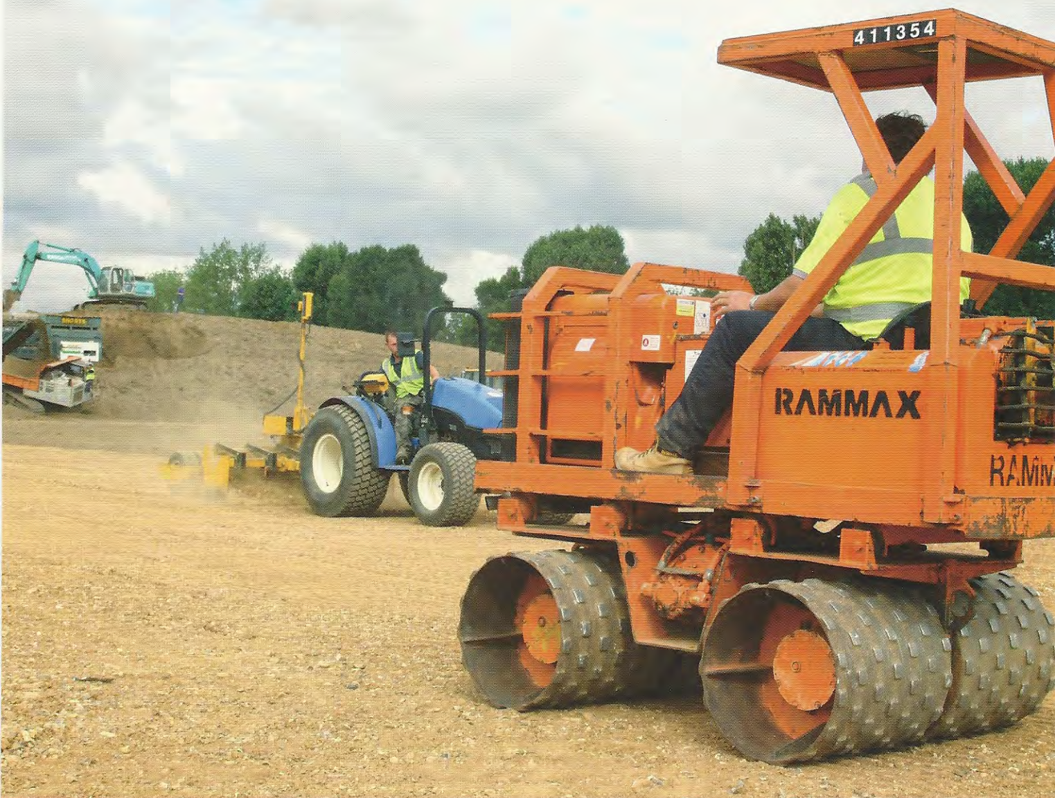
Opposite page: late July: a bird's eye view of the earthworks. Above: pressing the base of the cricket square prior to Surrey Loam application. Rigby Taylor's R9 was used for seeding
